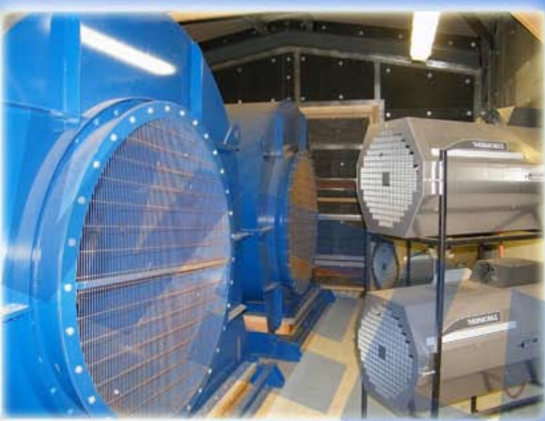
2x75hp units complete with burners.
